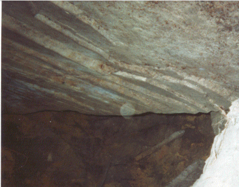
Section 3: This picture indicates that whoever cut the sandstone, had to come from below. Hewn sandstone roof of underground chamber facing South south west. © 2001 v. Senff
