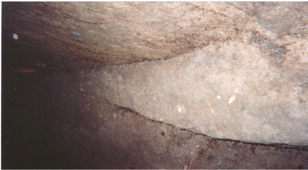
West wall [bottom] made of local sandstone and hewn roof of underground chamber. © 2001 H - D von Senff
